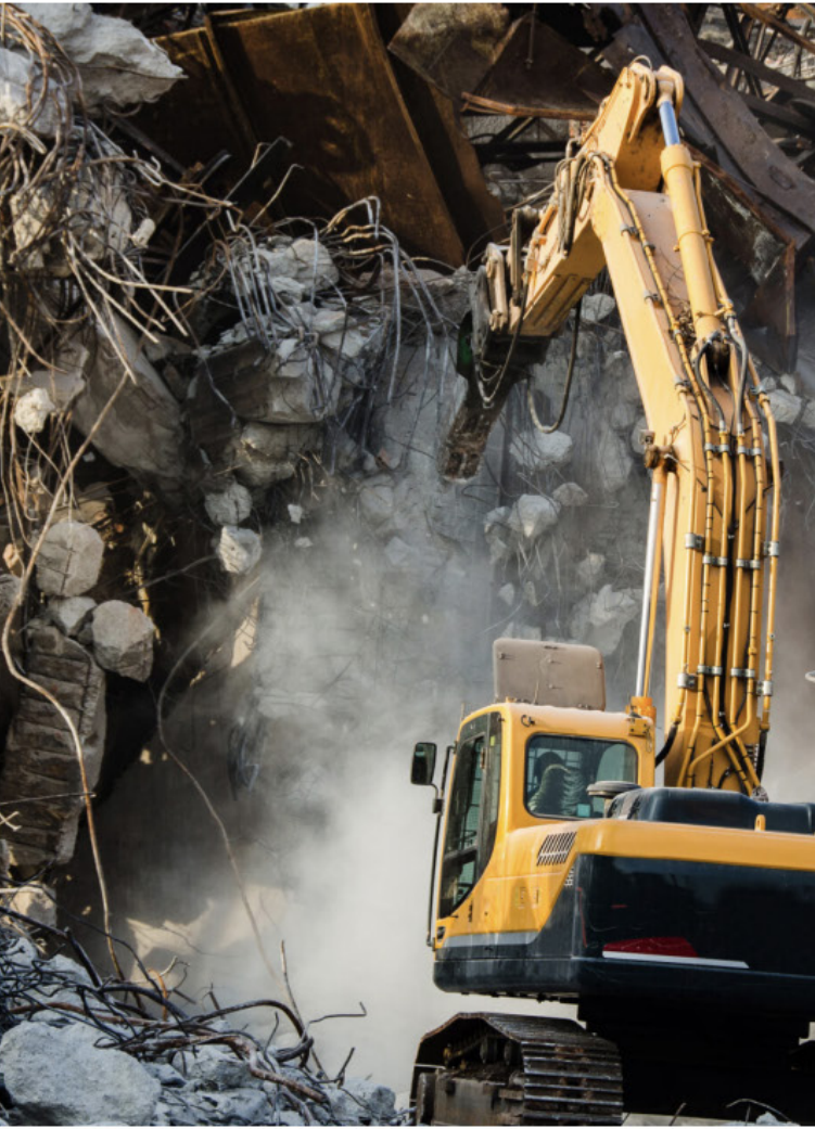
Demolition of a reinforced concrete frame building
